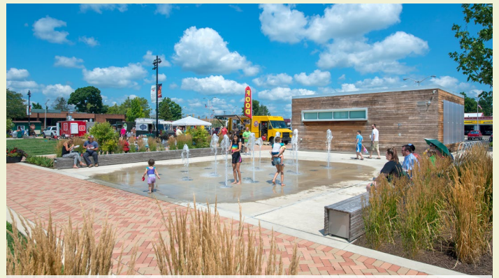
Spray Plaza and Restroom Building at Jack Elstro Plaza
