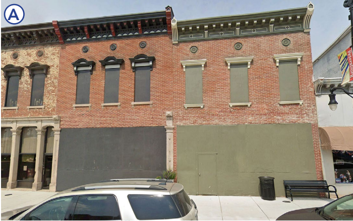
606 & 608 Main Street - Facade
