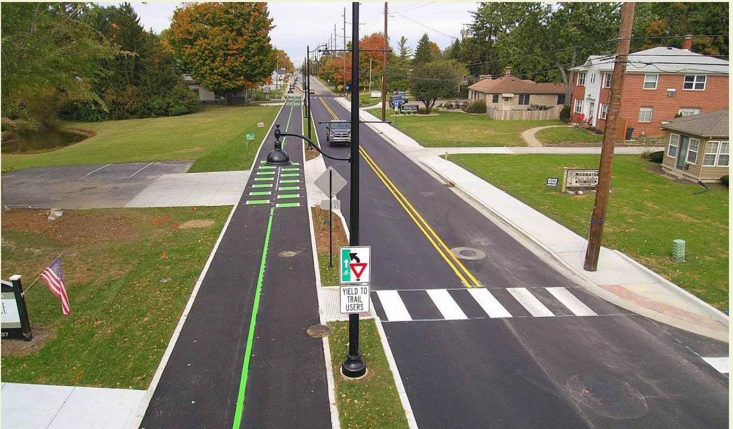
Aerial View of Greenwood Madison Avenue Complete Street Project
