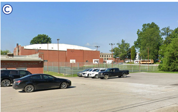
Administration Building and Parking Lot
